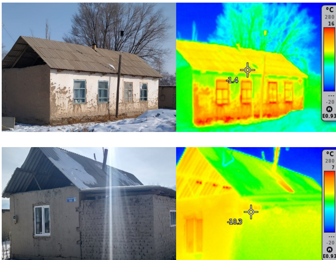
Fig. 3 Thermal images of uninsulated Kyrgyz houses in Ak-Tal region during the heating season
