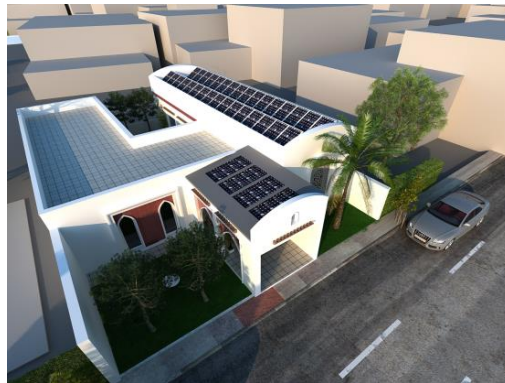
Fig. 2: The typical residential building under study
