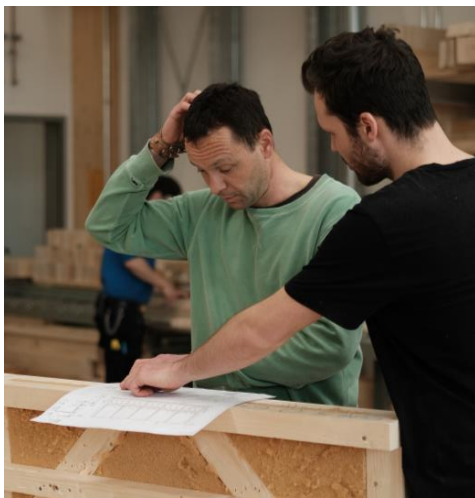
Figure 13: Some difficult connections were solved during prefabrication.
