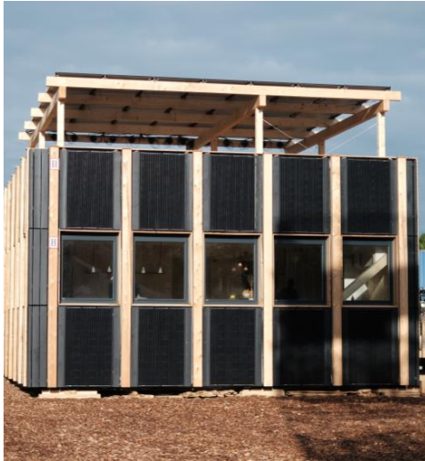
Figure 9: Eastern and southern facade of the HDU are solar activated with PVT modules
