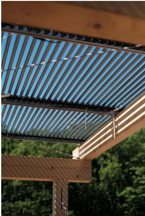
Figure 7: Air- and water-permeable solar roof with solar tubes for energy generation
