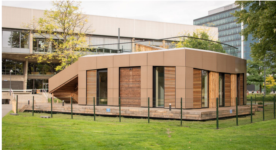
Fig. 6: A picture of the RDU during test-building in July 2021 at the campus of the Eindhoven University of technology.
