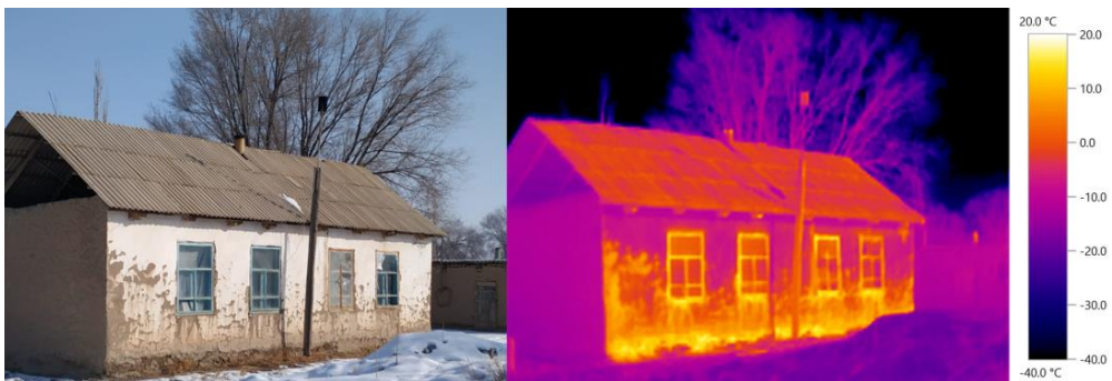
Fig. 3: Thermography of a typical rural house
