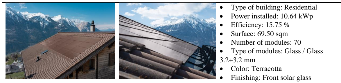
Fig. 7. Erschmatt project, Switzerland: overview of the solar façade (left) and BIPV modules' detail (in the center). On the right: project's figures. Images courtesy of SUNAGE
