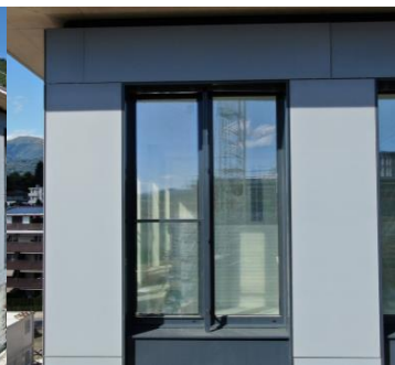
Fig. 4. Pregassona project, Switzerland: overview of the solar façade (left) and BIPV modules' detail (in the center). On the right: project's figures. Images courtesy of SUNAGE
