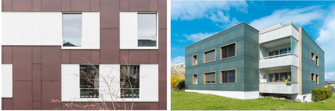
Fig. 2. Examples of modules' size customization for adapting the BIPV system to the façade geometry. On the left; Wohnüberbauung Männedorf Project, Männedorf, Switzerland (2020-2021) on the right: Opfikon Project, Opfikon, Switzerland (2018). Images courtesy of SUNAGE sa.
