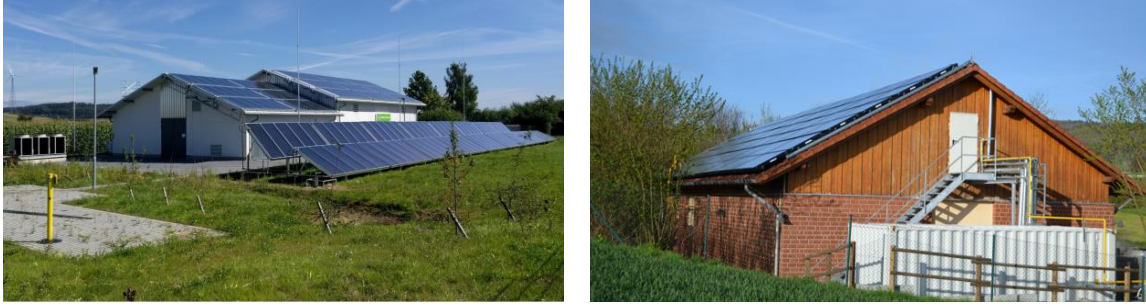
Fig. 1: Pictures of the GPRMS Ostheim with a 295 kW th SHIP plant and 123 kW th GAHP (left) and the GPRMS Neu-Eichenberg with a 95 kW th SHIP plant and 123 kW th GAHP (right).
