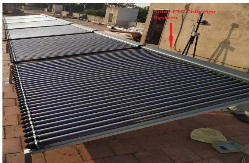
Fig. 5: Solar thermal evacuated tube collector system
