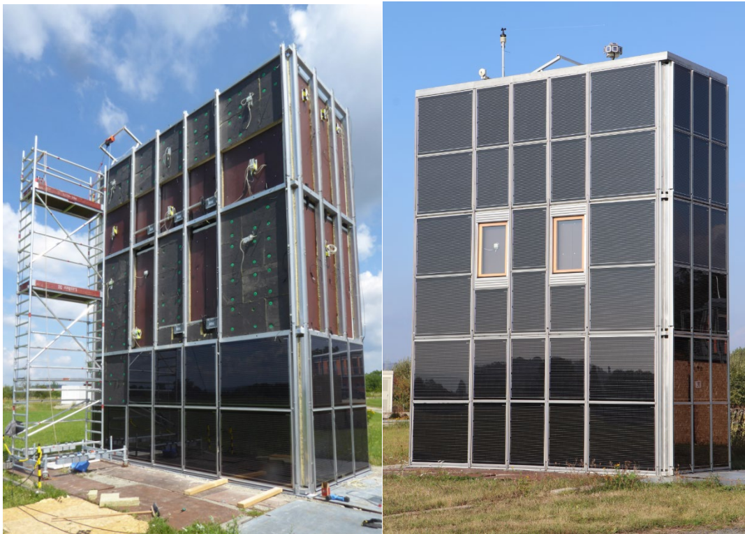
Fig. 6: Left: Test facade during assembly (left) and after finalization (right).
