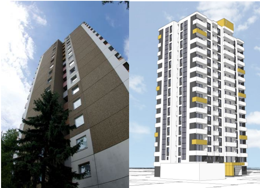
Fig. 1: Left: View of the façade of the demonstration building in Frankfurt foreseen for the installation of two strips PV. Right: CAD-Model visualizing the planned PV-strips (ABG)
