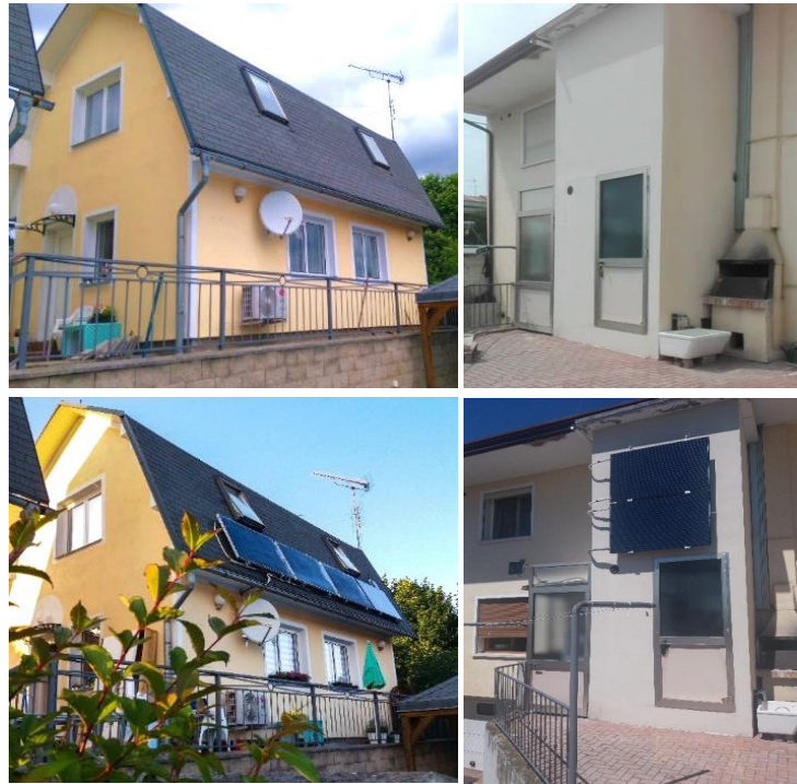
Fig. 2: The single-family house considered for the test previous (up) and post intervention (down), located at Jablonec nad Nisou (50.7N, 15.1W coordinates, left) and San Martino di Lupari (45°38'N, 11°51'W coordinates, right).
