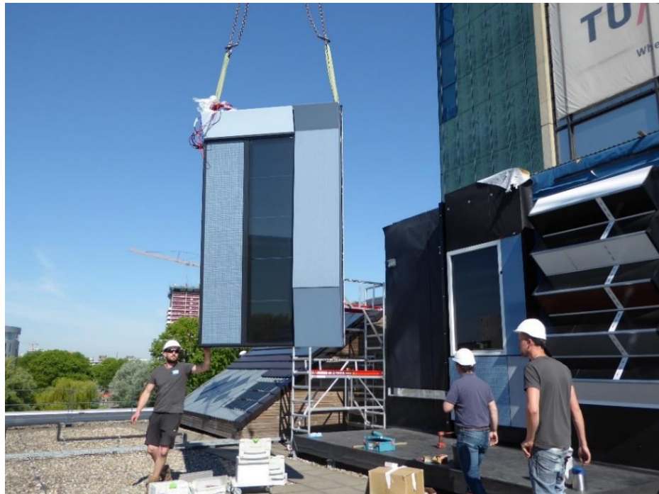
Fig. 2: Installation of a PREFAB element
