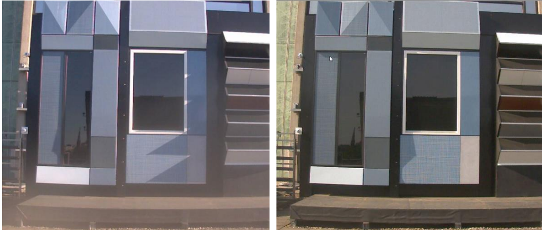
Figure 5: Left: Shade patterns in the morning of the 17 th of April of 2022 caused by the neighbouring PV setup (ZigZag) Right: Shade on panel D, caused by the protruding part of panel C2 in the afternoon of the 17 th of April 2022.
