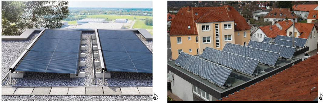
Fig. 4: Evacuated tube collector lying flat on the roof (left, © Viessmann GmbH) and solar thermal system with orientation parallel to building's edges (right, © Ritter Energie- und Umwelttechnik GmbH & Co. KG)
