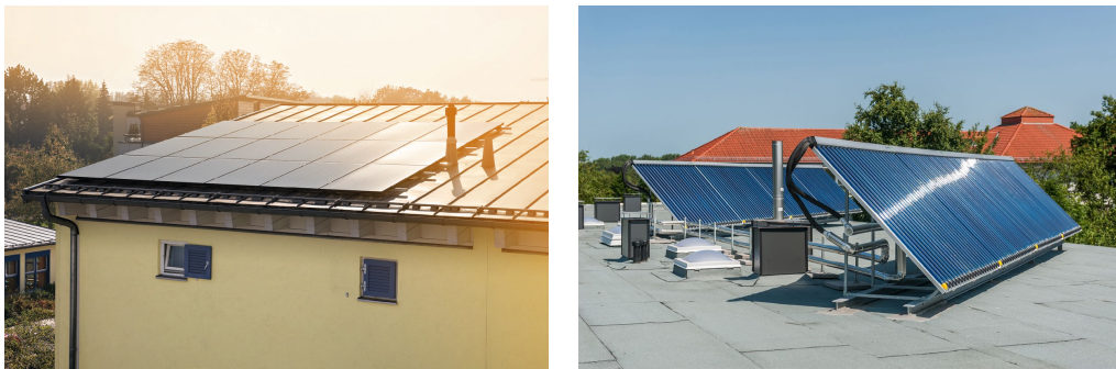
Fig. 6: Reflection of sunlight on photovoltaic modules (left, © SOLARWATT GmbH) and solar thermal collectors (right, © Ritter Energie- und Umwelttechnik GmbH & Co. KG)
