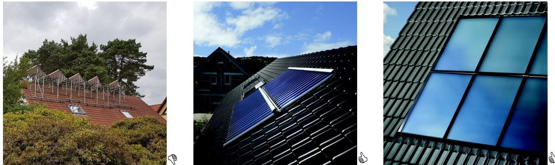
Fig. 2: Elevated photovoltaic modules (left, © Felsmann), roof-parallel evacuated tube collector (center, © Vaillant GmbH) and in-roof flat-plate collector (right, © Vaillant GmbH)
