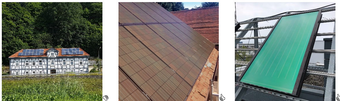
Fig. 3: High color contrast between roof and PV modules (left, © Felsmann), red photovoltaic on red roof (center, © BISOL Production Ltd.) and green solar thermal collector developed by Fraunhofer ISE (right, © Fraunhofer ISE (Andreas Wessels))
