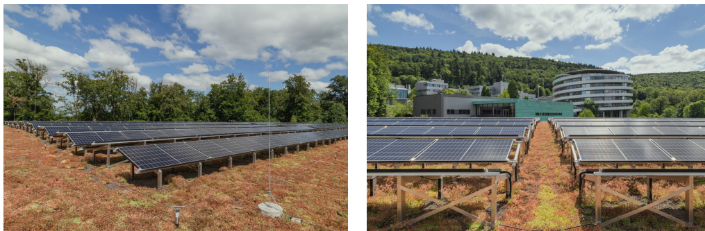
Fig. 5: Showcase combination of photovoltaic and green roof (© Optigrün)
