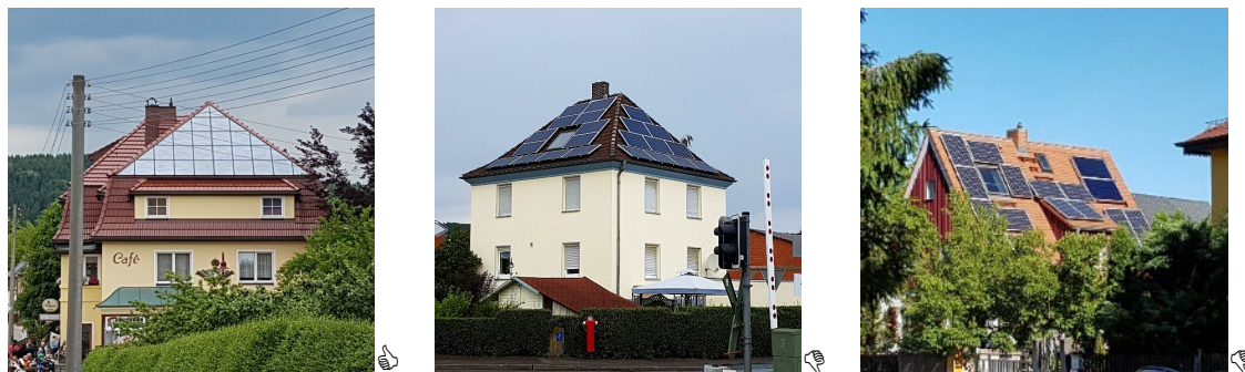
Fig. 1: Examples for photovoltaic area matching the roof shape (left, © Felsmann) and zigzag arrangement (center, © Felsmann), further a combination of horizontal and vertical PV modules and solar thermal collectors (right, © Felsmann)
