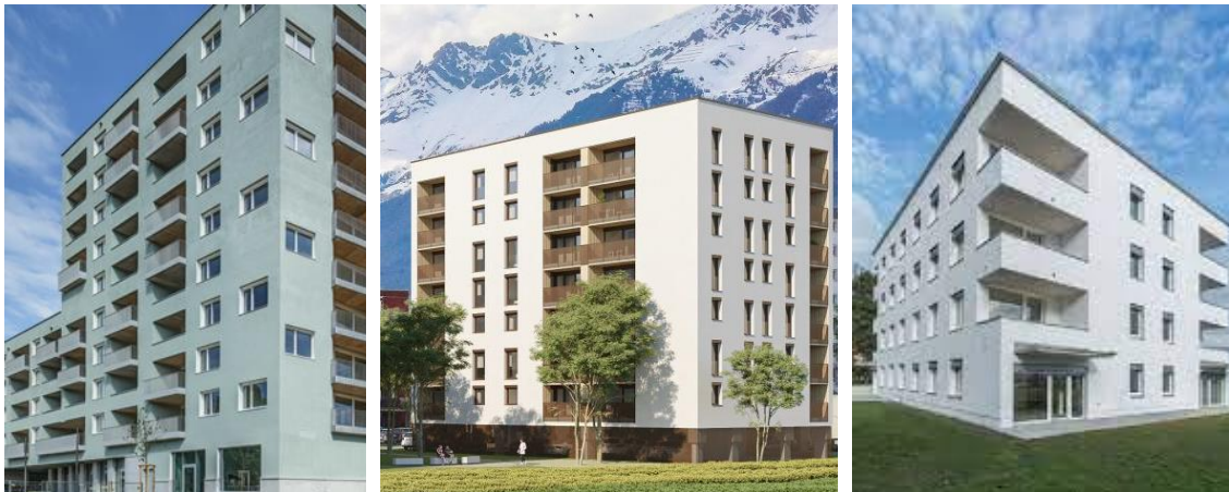
Campagne (NHT), Passive House with District Heating for DHW and GW-HP for SH and PV
