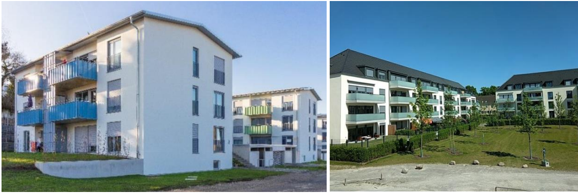
Fig. 4: Cluster of multi-family buildings in Konstanz (left) [source: WOBAK] and Wolfsburg (right), DE
