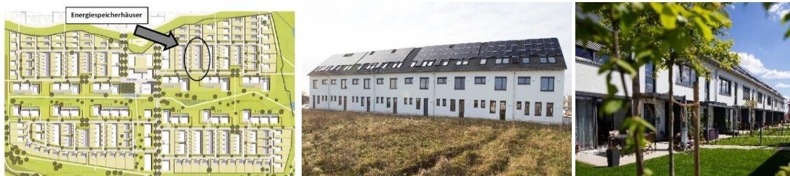
Fig. 2: Building cluster Herzo Base, Herzogenaurach, DE
