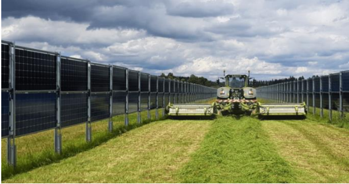
Fig. 2: Example of an bifacial Agri-PV system. (Next2Sun GmbH, 2022). The distance between the module rows is chosen in such a way that the agricultural machine has enough space to mow the field and thus cultivate the area.
