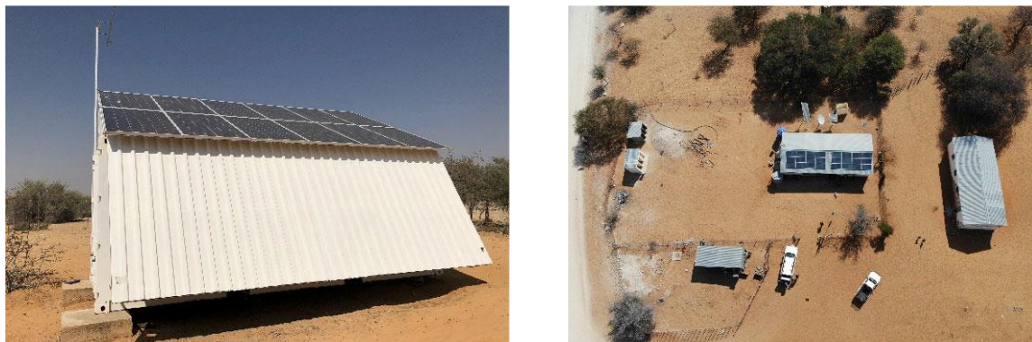
Fig. 2: Containerized and rooftop PV systems at the veterinary centre and school in Utsathima (source: author)
