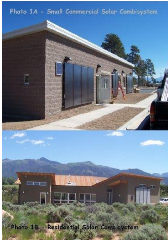
Photo 1: Examples of Small Commercial and Residential Solar Hydronic Combisystems.
