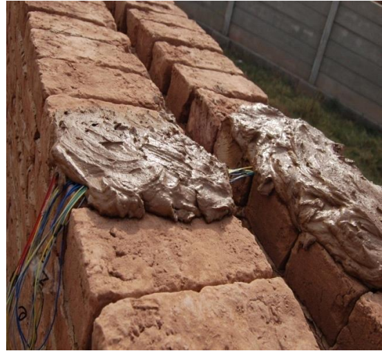
Fig. 8: Temperature sensors embedded in adobe wall
