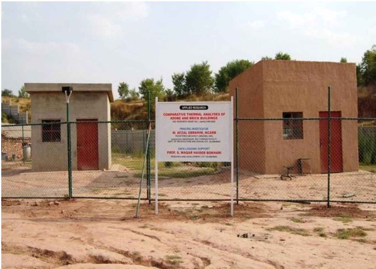
Fig. 6: Brick building and (left) and adobe building (right) constructed side by side on site for testing
