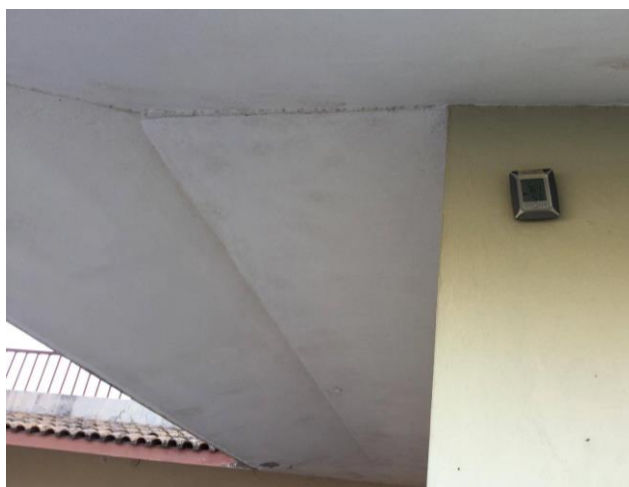
Fig. 8: Sensor module monitoring outside air and relative humidity
