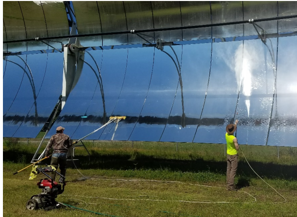
Figure 5. Mirror Washing Procedure
