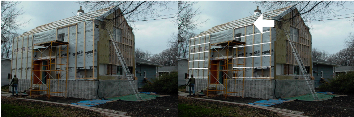
Fig. 9: Completing the crisscrossing lattice system for ventilation on façade
