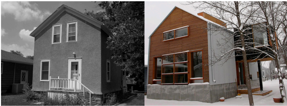
Fig. 2: Original dwelling and refurbished dwelling
