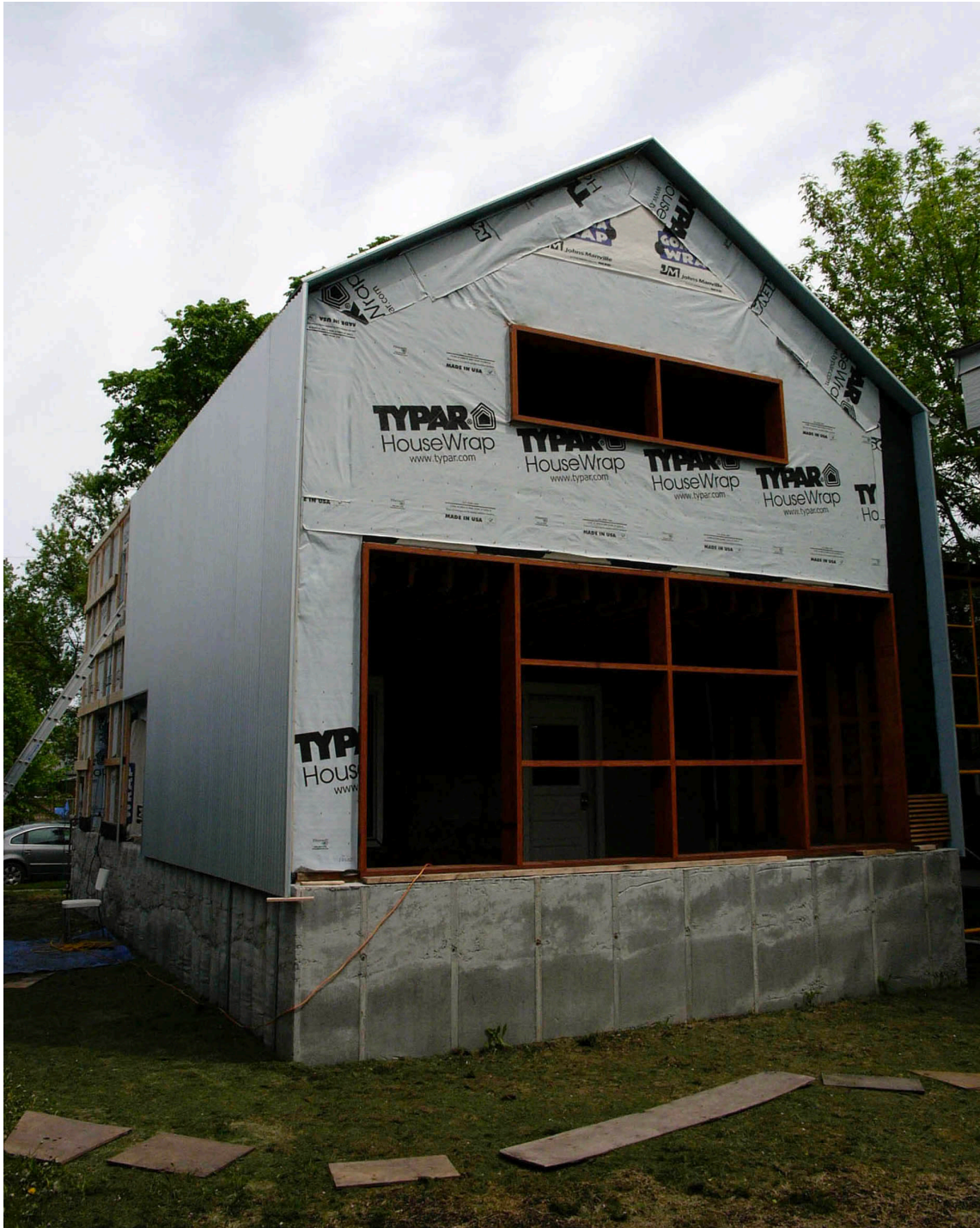
Fig. 11: Galvalume, crisscrossing lattice system, weather-resistant barrier
