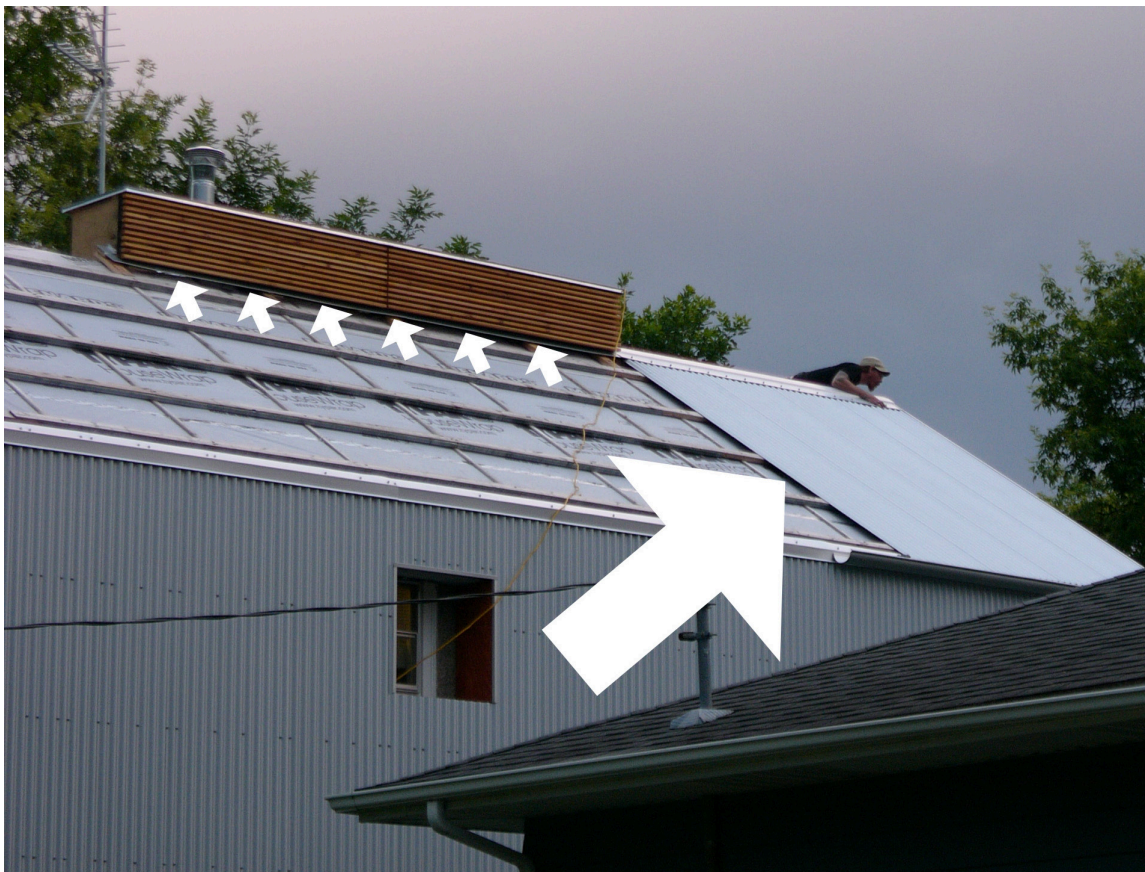
Fig. 10: Completing the crisscrossing lattice system for ventilation on roof
