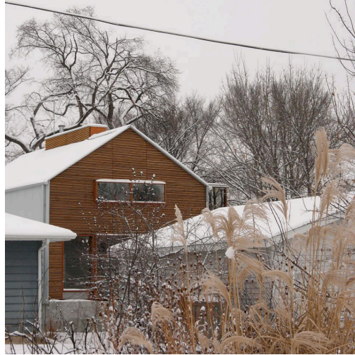
Fig. 14: Upgraded south façade – House in a House
