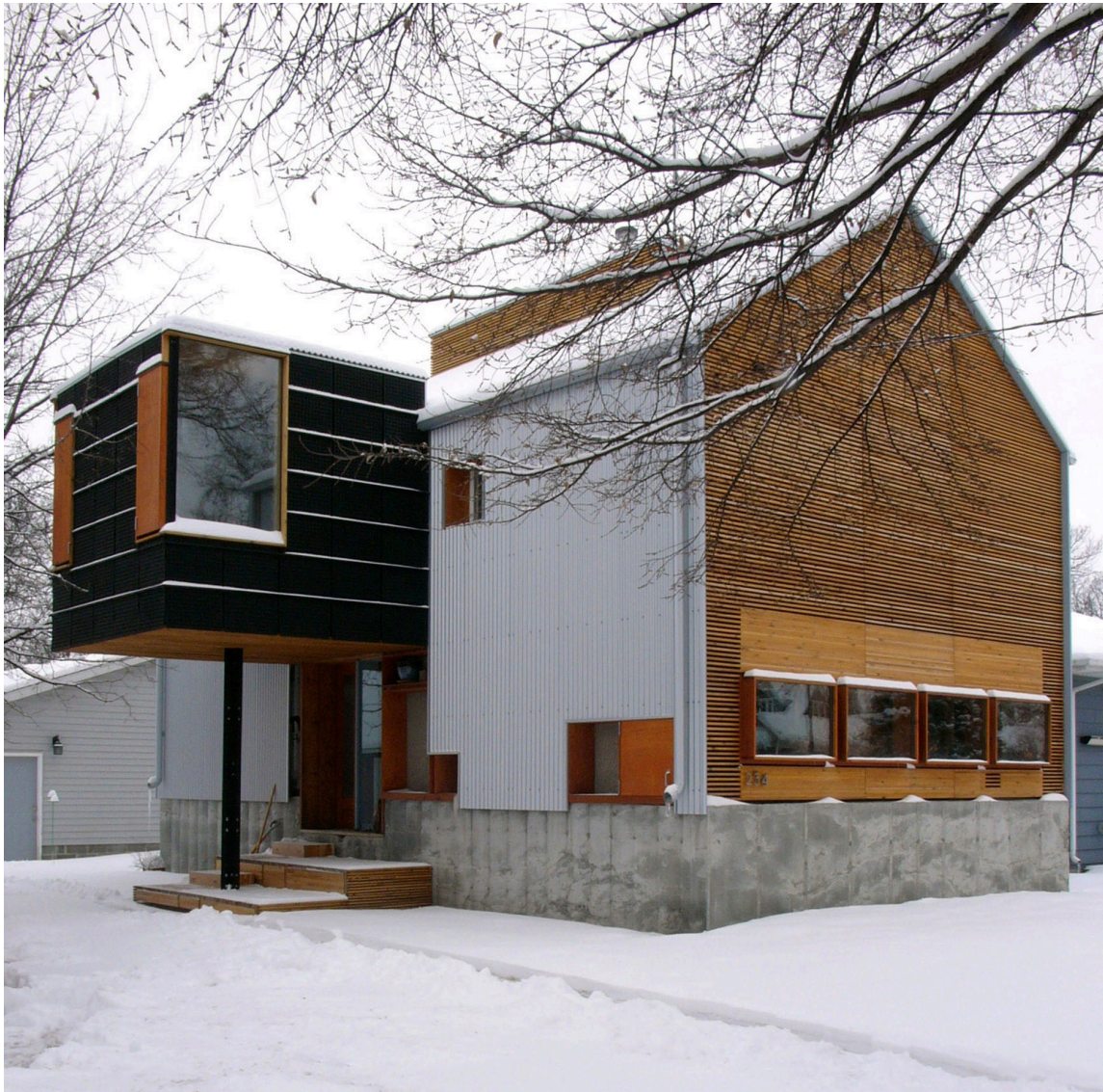
Fig. 13: The retrofitted dwelling seen from the northeast corner
