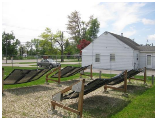
Absent are metal post, beams, stringers, and concrete
