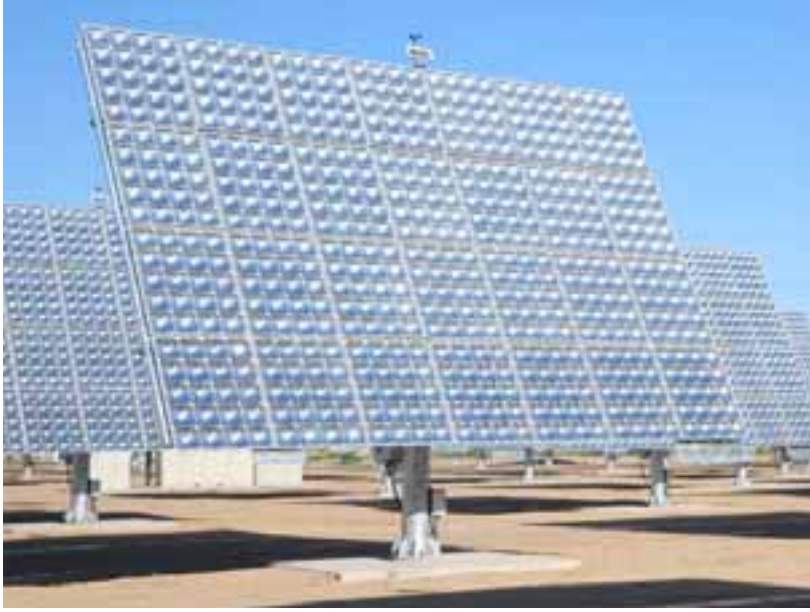
Fig. 2. Example of CPV deployment of aplanatic optic concentrators. The large number of modules on each tracker require accurate alignment of the individual modules and a stiff construction to have each element pointing in the same direction (SolFocus, 2010).
