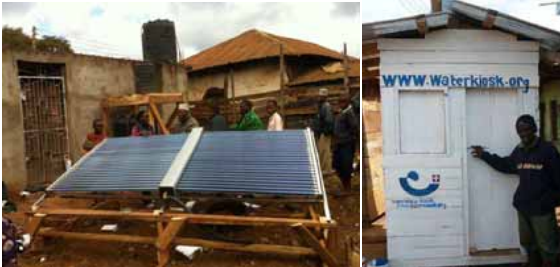
Fig. 9: In the left picture the SoWaDis system in the village of Lukozi/Tanzania is shown that was set up in August 2011. On the right hand side, the SwissWaterKiosk hut for selling the purified water is shown.
