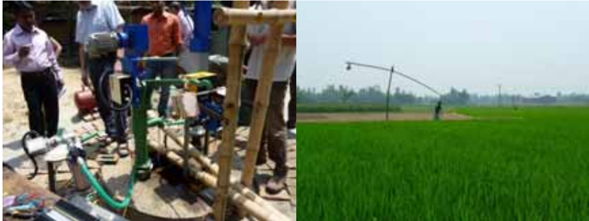
Fig. 5: Swiss Solar Water Pump developed at BUAS Biel and implemented in Bogra, Bangladesh (left). Manually-operated water pump (right) in Bogra, Bangladesh (both photographs taken by I. Kunz and D. Tschanz on 10 and 6 April 2011).
