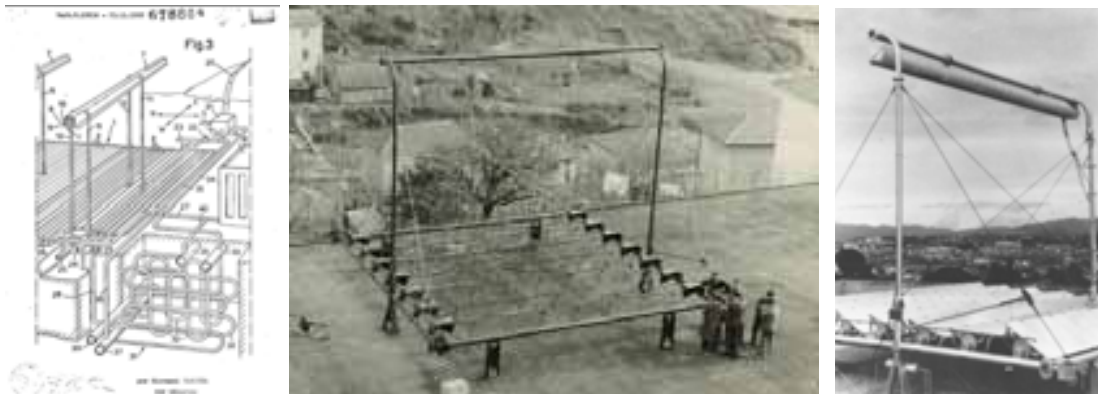
Fig. 7: World's first linear Fresnel concentration-type solar plant, built and tested at Marseilles (France) in 1963/1964. Left: drawing of the patented LFC; Right: Photos of Francia's first LFC prototype (Francia Archive, Museum of Industry and Work, MUSil, Brescia, Italy).
