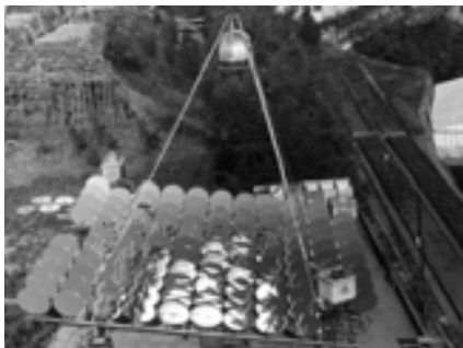
Fig. 10: Left: World’s first point-focus Fresnel reflector concentrator or solar tower, built and tested at Sant’Ilario, in the township of Nervi, near Genoa (Italy), in 1965 (Francia Archive, MUSil Brescia). Right: Francia’s solar tower patent filed in USA in 1966 (Digitized by Google).
