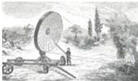
Fig. 4. A large burning mirror of the late 1700’s built in sections (Butti and Perlin, 1980)
