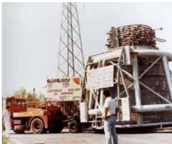
Fig. 12: Eurelios’ solar boiler before its installation on the top of the tower, photo 1980, MUsil, Brescia, Italy.
