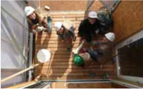
Fig.13: Prototype construction Campus Sant Cugat March 2011
