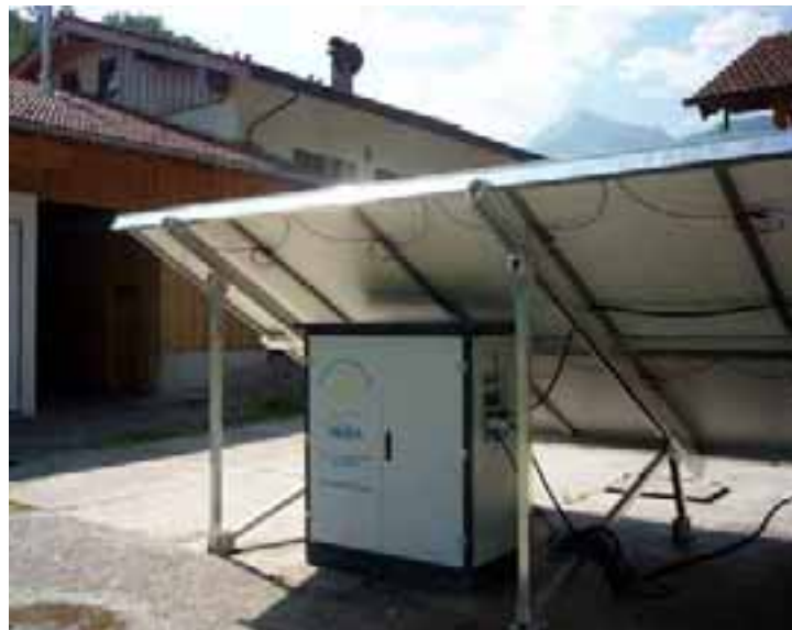
Fig. 2: PV-hybrid-CEB system supplying power for the one family house that is seen in the background
