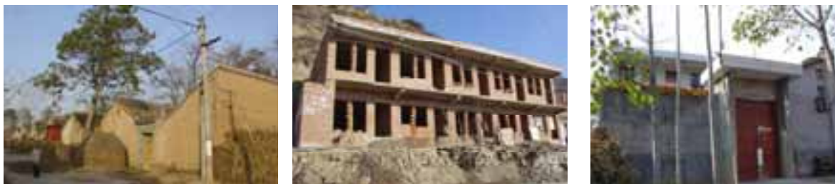
Fig 2 Heavy clay structures (left) replace by simple concrete and brick structures (mid and right)
