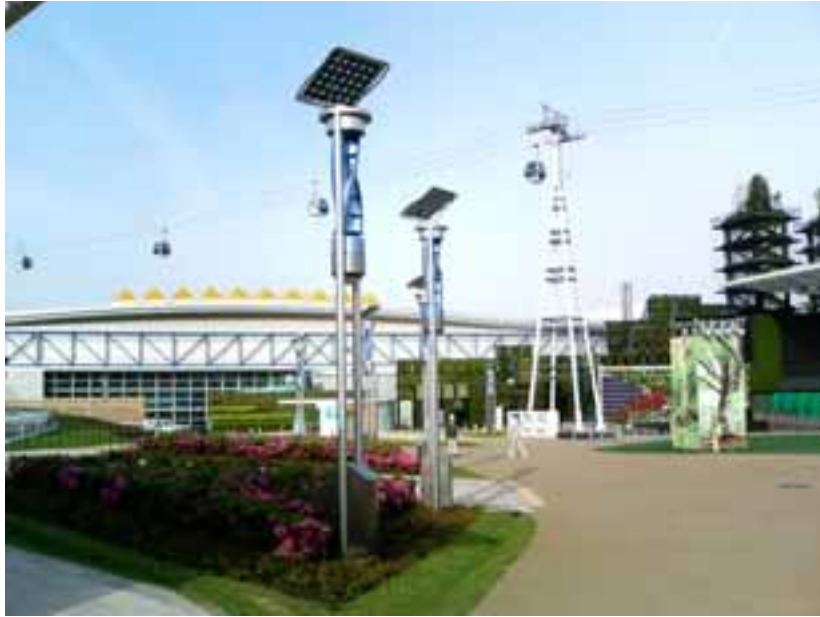
Fig. 5: Solar cells & wind turbine hybrid tower “Kaze Kamome” by Panasonic Ecology Systems Co., Ltd.
