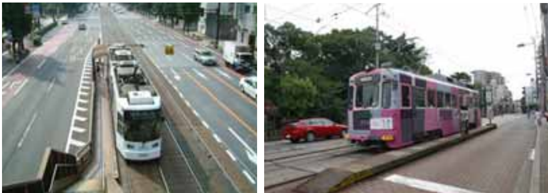
Fig. 3: Roofless platform and small roof platform for tram in Japan (left: Kumamoto / right: Osaka)
