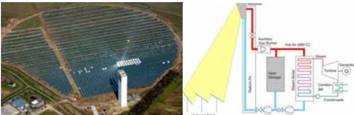
Fig. 1: Jülich solar central receiver plant (left) and plant layout (right)
