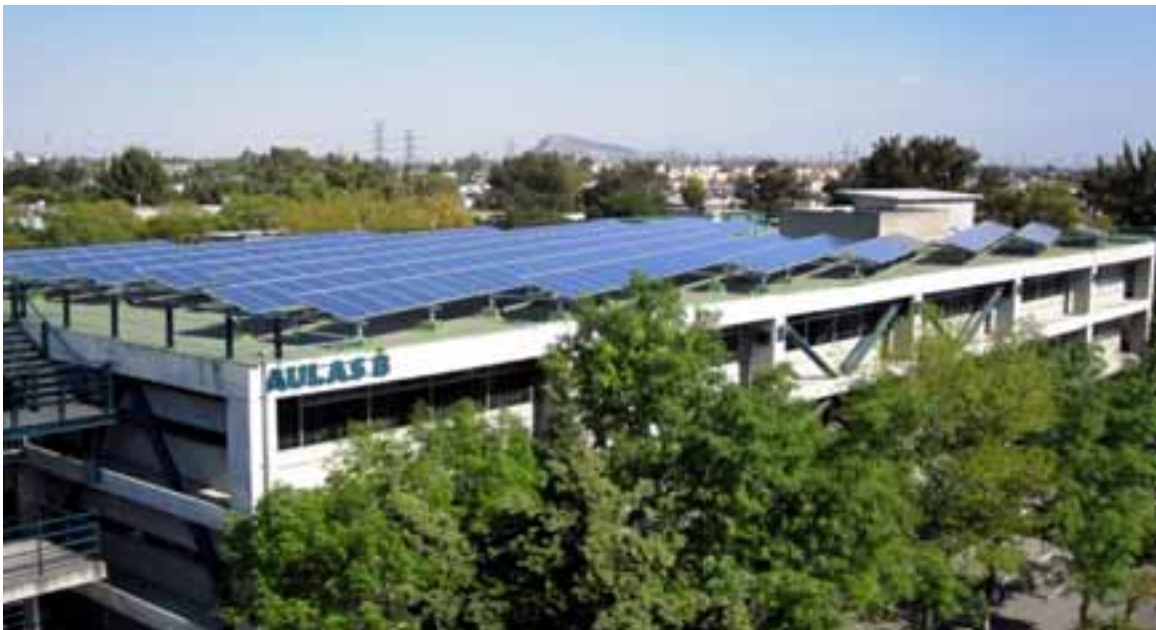
Figure 1. 60.06 kW p Photovoltaic System at the University Autonomous Metropolitan in Mexico City
