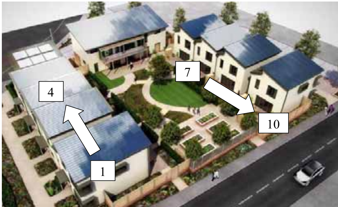
Figure 1 Greenwatt Way development. Houses are numbered clockwise from bottom left.
