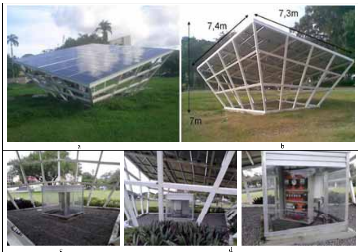
Fig. 1: Campus system - a) Front view, facing Geographic North, inclination ( \beta=22^\circ ); b) view looking South (without the box); c) the glass box in the sculpture interior; d) equipments in the box: inverter, data acquisition, and control instruments
