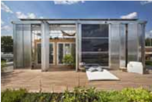
Fig.5: General view LOW3 south facade
