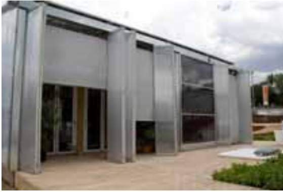
Fig 11: South façade open with shading device
