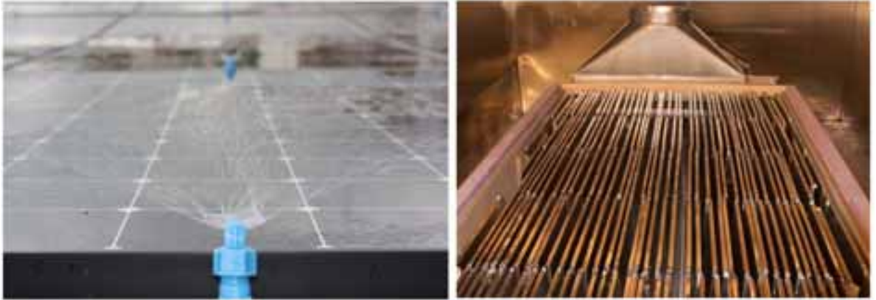
Fig. 5: Passive radiation cooling on the roof using the PV panels and the PCM channel.
