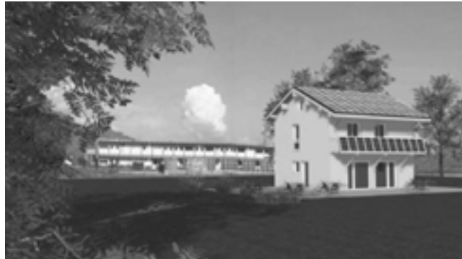
Fig. 2: View of the South and East façades of the INCAS house
