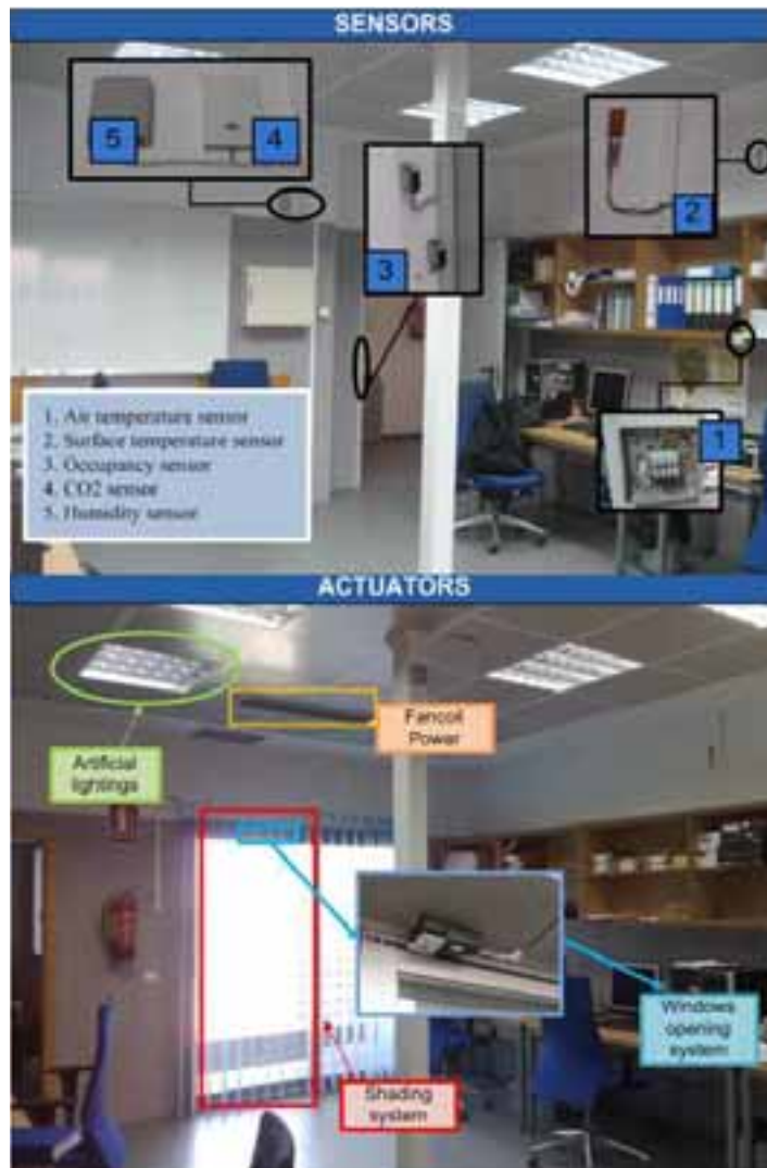
Fig. 2: Sensors and actuators in a typical office
