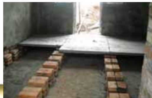
Fig. 22 Space layer in construction (photo by Wei Luo)
