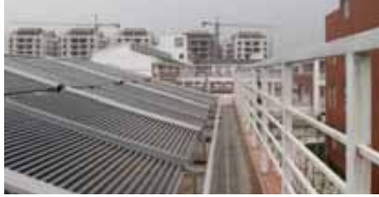
Fig. 23 Heat collectors on canteen's roof (photo by Wei Luo)
