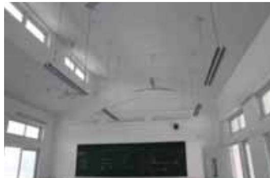
Fig. 20 Classroom with clerestories (photo by Wei Luo)
