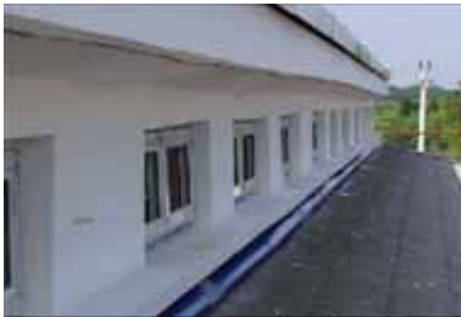
Fig. 19 Clerestories of classrooms (photo by Wei Luo)
