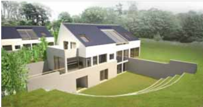
Figure 1: Z-en House South-west Façade (Source: MEARU Mackintosh School of Architecture)
