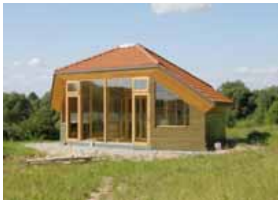
Fig. 5: The view of the built house. Photo by JSK Ecococon
