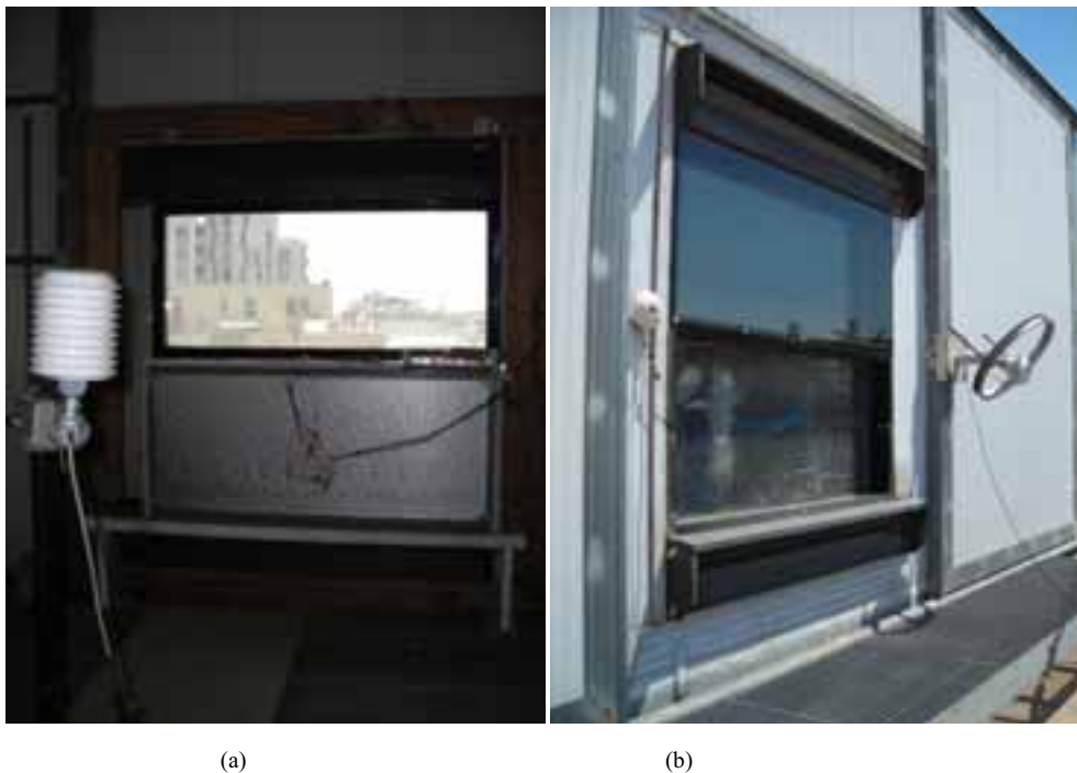
Fig. 4: indoor (a) and outdoor (b) view of the multi-functional façade element
