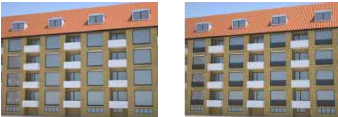
Fig. 3: Illustration of renovation solution 3 with increased window area and the dynamic parapet inactive (left) and active (right)
