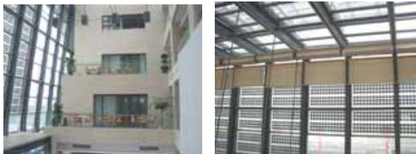
Fig. 4 Atrium Lighting and Shading
