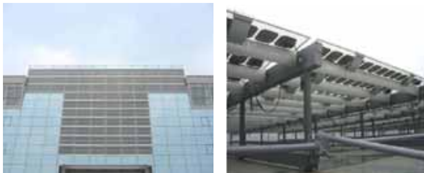
Fig. 2 PV Façade and Rooftop Installation
