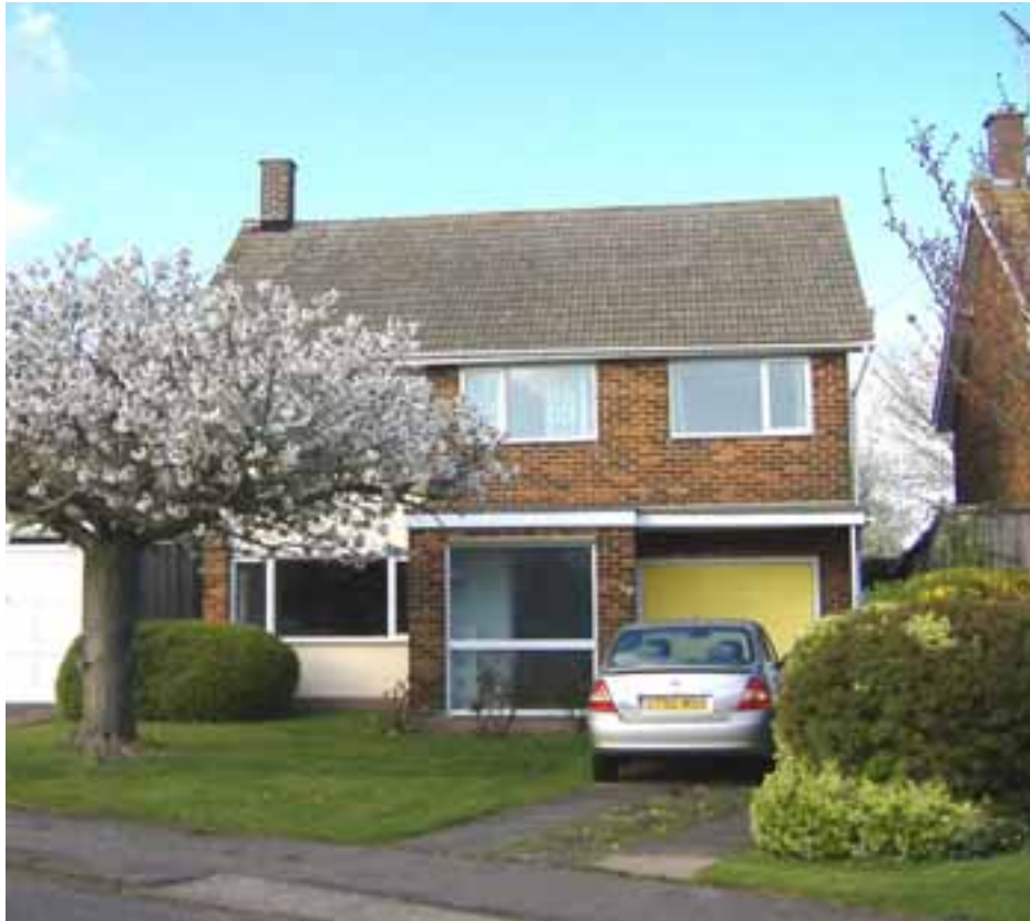
Fig. 1: The test house.
