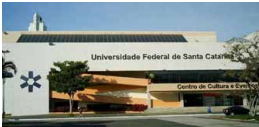
Fig. 1: Flat, latitude-tilted ( 27^\circ ), north-oriented, 10.24 kWp building-applied PV generator installed on the rooftop of the Universidade Federal de Santa Catarina (UFSC) theatre main building.
