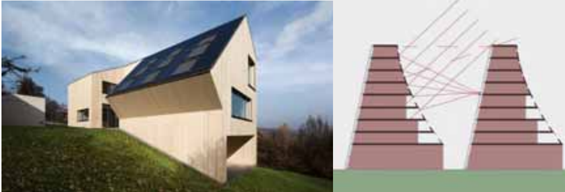
Fig. 8: Examples of "technomorph" forms in relation to the use of photovoltaics. (left) Sunlight House II, Henry Troy Architect, (right) Building integration of stationary reflectors with PV or PVT absorbers tracking. Architectural concept of buildings with integrated systems PVT in combination with reflectors for lighting the interior (Cisbat Congress 2009)
