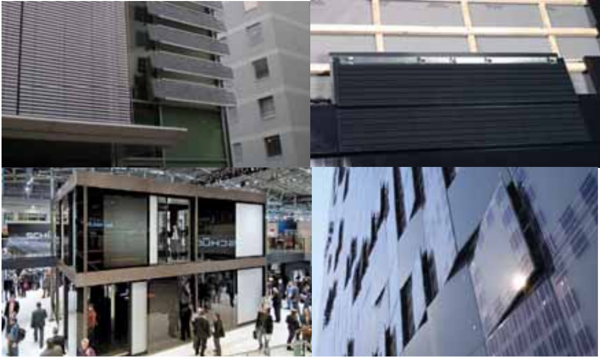
Fig. 8: Different principles of technological innovation of BiPV systems: (top left) The PV as a added body. Oskar Von Miller Forum, Thomas Herzog+Partner, Monaco (photo author); (top right) Example of stratification of roof with basic photovoltaic building elements that replace the traditional roof covering. Creaton AG “Solesia”; (bottom left) Intelligent facade Schueco Energy 2 at BAU 2009 in Monaco; (bottom right) “Green Pix Zero Energy Media Wall” in Beijing (China), Simone Giostra & Partners Architects + Arup Engineering, 2008.
