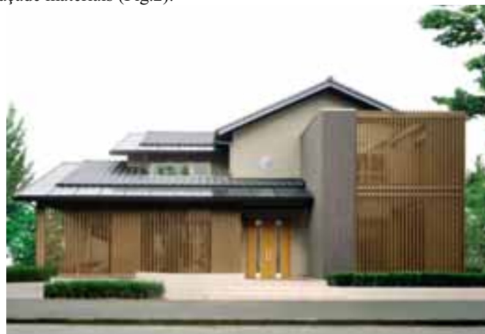
Fig. 2: ‘Wa no Nagomi’ zero energy cost house in Japan (Source: SANYO Homes Corp.)
