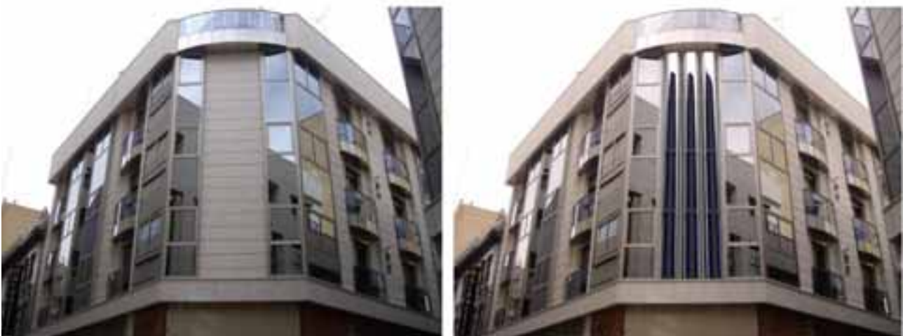
Figure 2: Photographic editing of an installation of curved collectors in a real facade
