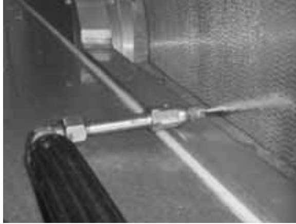
Fig. 7: Cleaning of the heat recovery wheel in May 2010
